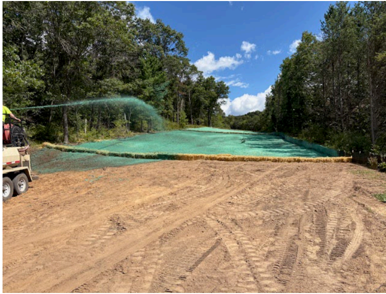
Facing east near MP 2.3, American Hydro Seed hydroseeding slope
