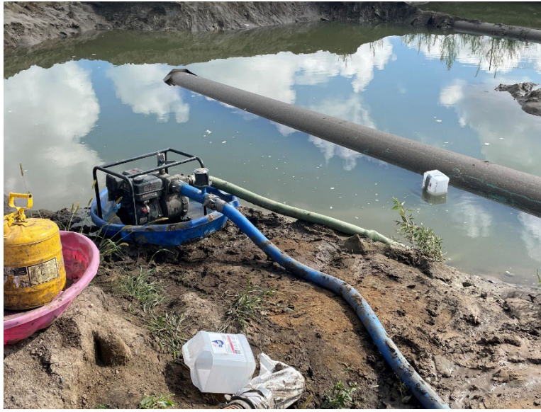
Facing southwest at MP 31.35, K&K utilizing an empty jug to suspend suction intake while dewatering
