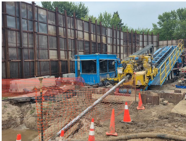
Facing west at HDD P4-5, reaming completed
