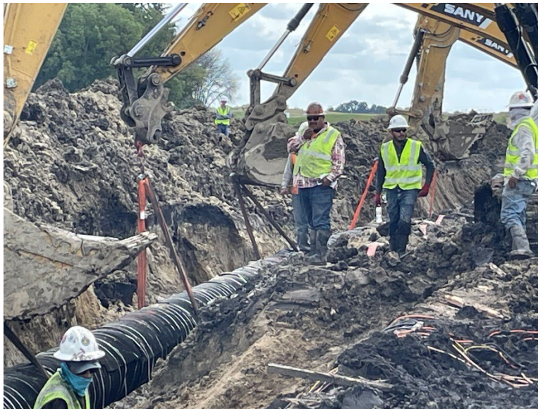
Facing southeast at MP 31.7, K&K lowering-in mainline pipe south of 140th Street
