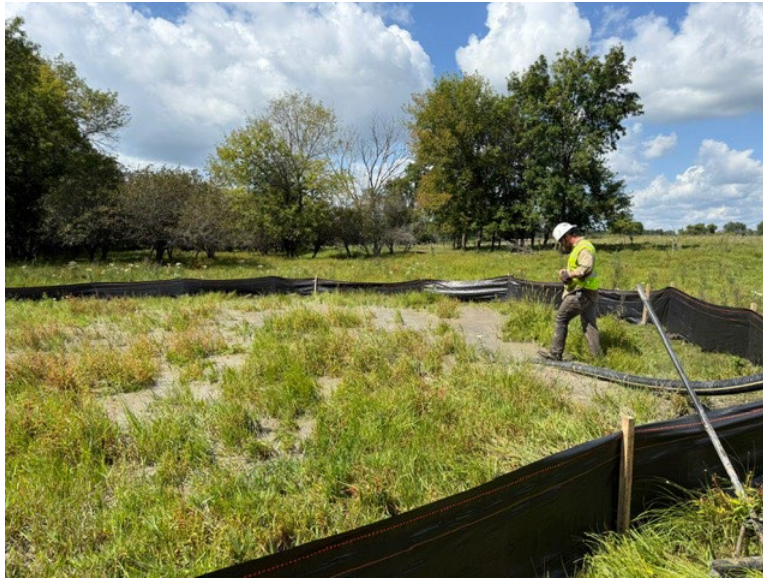
Facing west at MP 2.93, view of North Country containing and cleaning the IR on HDD P4-1 in wetland FRM-W01
