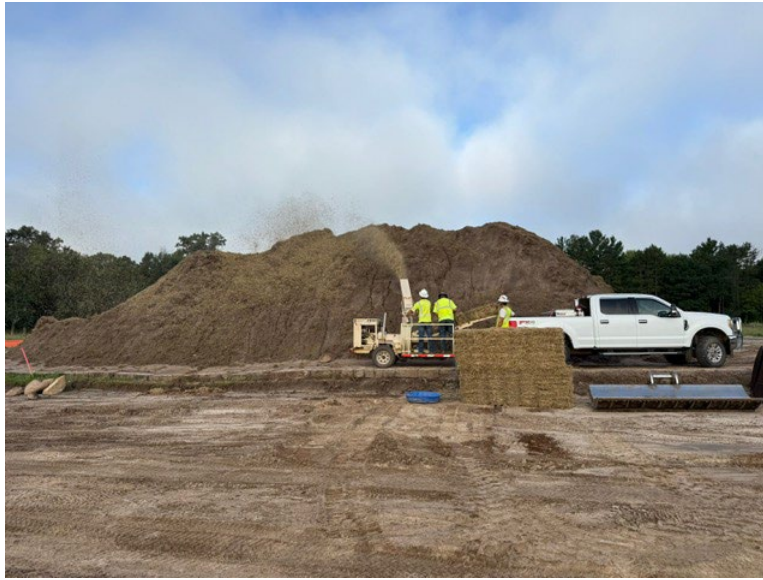
Facing west at MP 0.60, view of Otis stabilizing topsoil stockpiles
