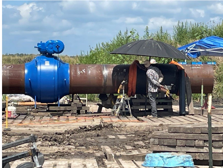
Facing north at MP 34.2, K&K fabricating tie-in piping
