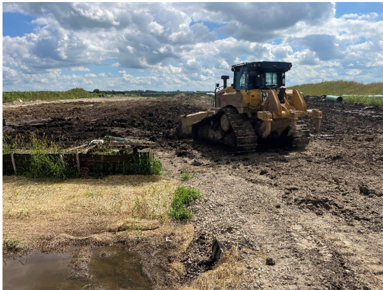
Facing south at MP 34.1, K&K utilizing a dozer to dry ROW and bring subsoil to grade
