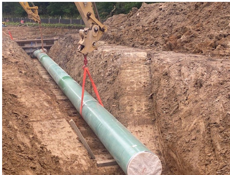
Facing east near MP 1.69, lowering-in ongoing
