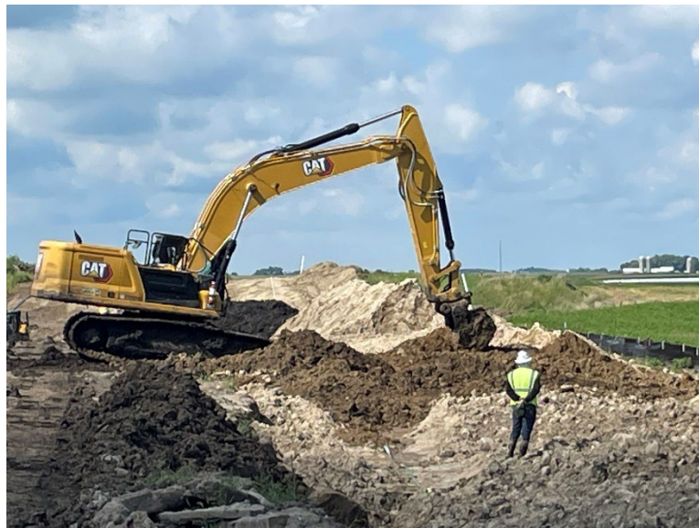
Facing north at MP 33.3, K&K backfilling trench north of County Road 80/154th Street
