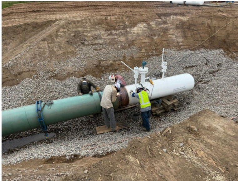
Facing east at MP 0.16, view of Otis installing the test header in preparation for testing the 30-inch-diameter pipe in the Hugo compressor station
