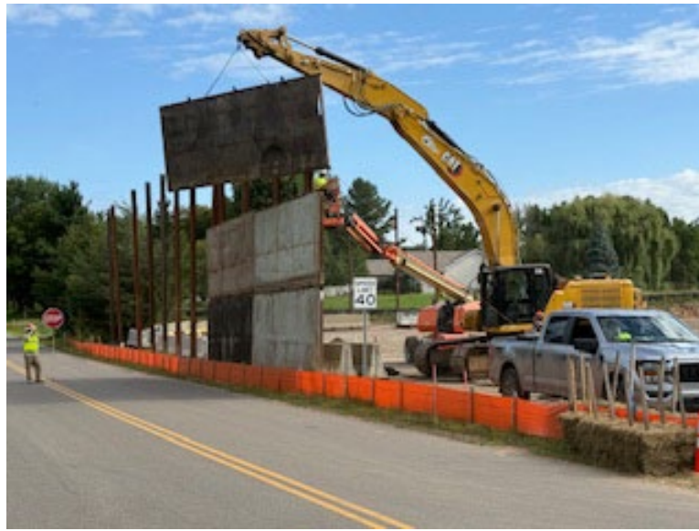
Facing north at HDD P4-1, sound wall installation being completed
