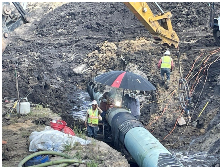
Facing north at MP 31.51, K&K completing mainline trench tie-in north of County Road 9/135th Street
