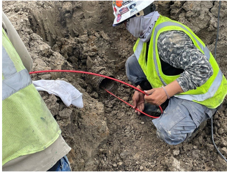
Facing southeast at MP 31.18, K&K utilizing a camera to scope damaged drain tile south of County Road 80/154th Street
