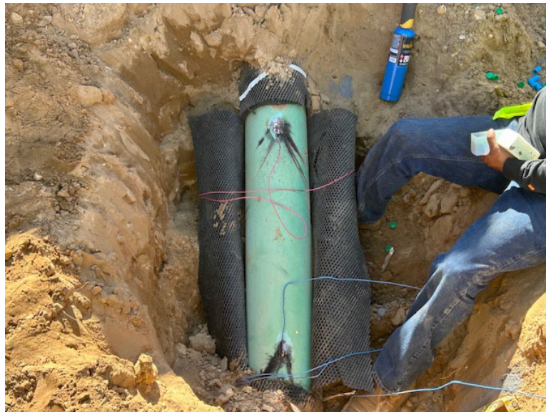
Facing east near MP 3.5, K&K installing test leads
