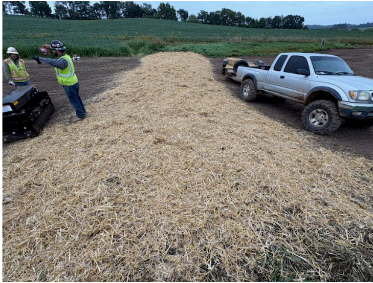
Facing north near MP 3.35, K&K seeded and mulched field berm
