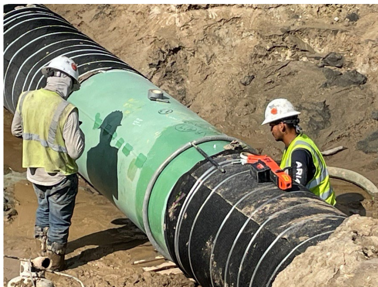
Facing northeast at MP 33.5, K&K repairing detected mainline holidays
