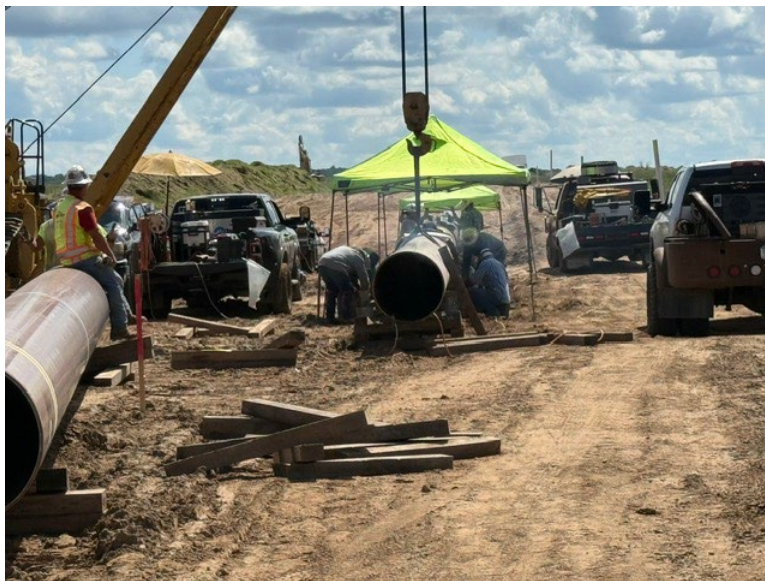
Facing south at MP 1.15, view of Otis welding bore pipe for HDD P4-2
