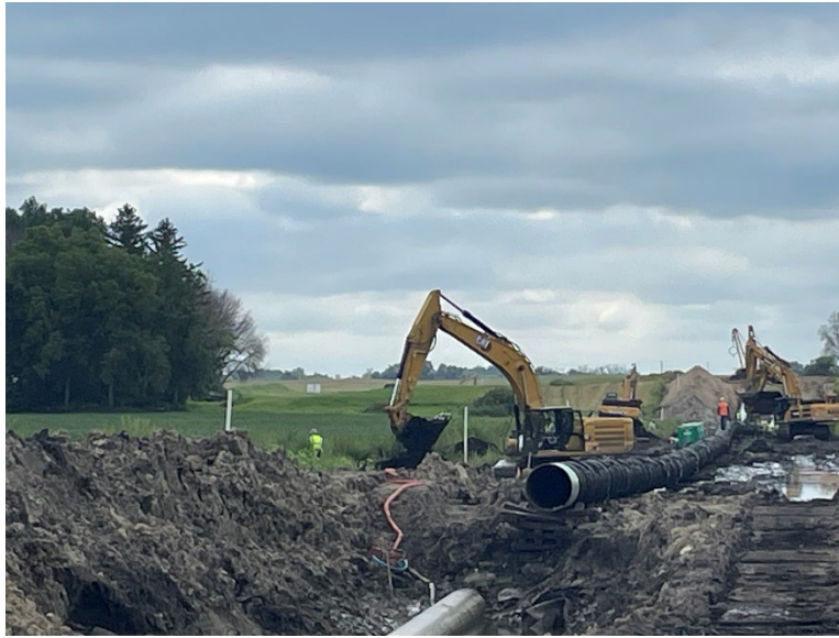
Facing south at MP 31.65, K&K utilizing a track hoe to remove topsoil from over D-line south of County Highway 9/135th Street
