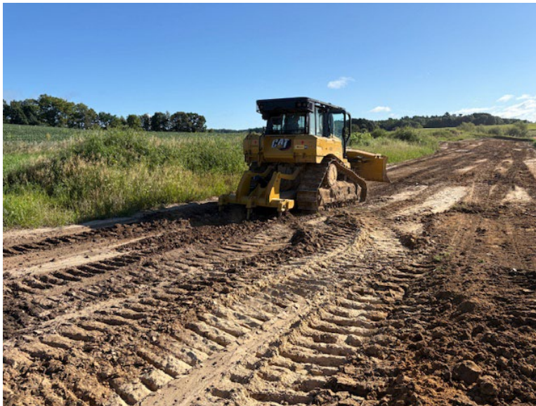
Facing east near MP 3.35, K&K decompacting subsoil in agricultural field
