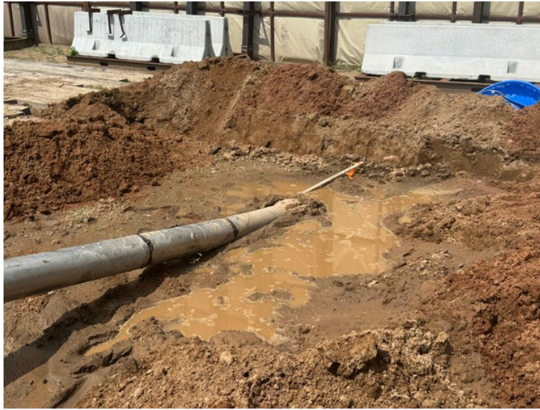
Facing north at MP 0.5, view of North Country commencing the pilot hole on HDD P4-1
